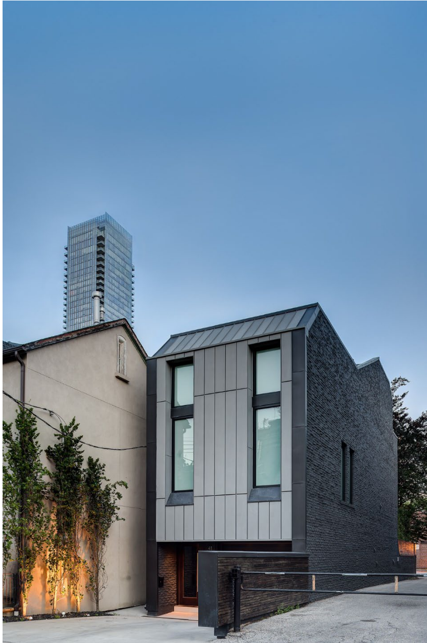
The new zinc exterior is a far cry from '70s-era beige siding. The dip in the roof informs the shape and size of multiple skylights. Contractor: GreenGold Construction Ltd.
